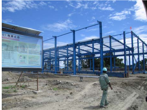
Infrastructure Construction at Plant Site
