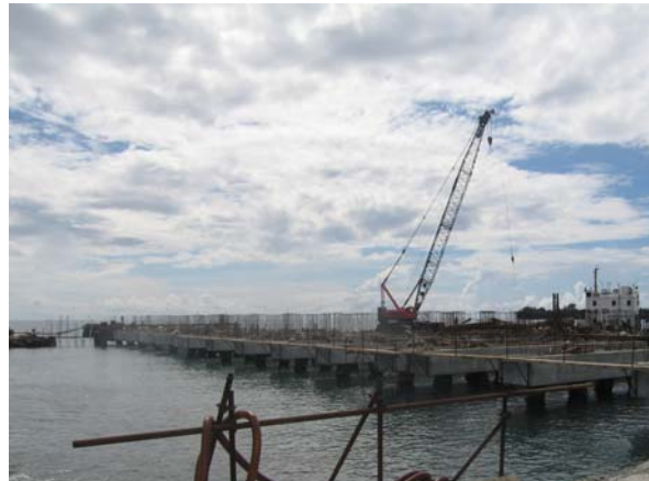
Basamuk Deep Water Wharf
