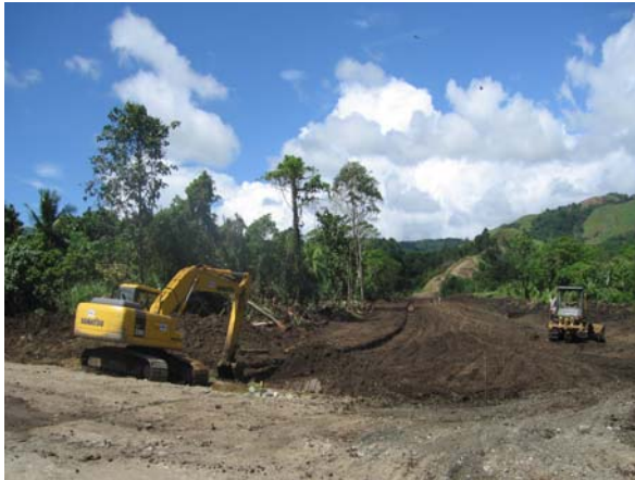
Construction of Road to Limestone Quarry
