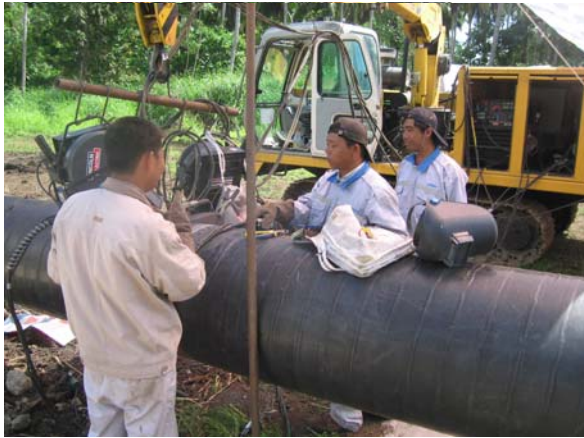
Installation of the 135km Slurry Pipeline
