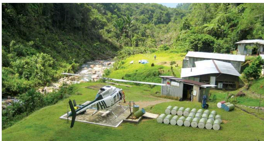
Frieda River Project base camp
