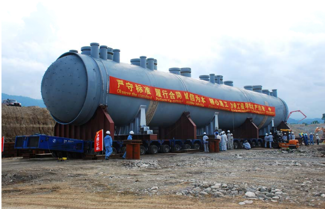
Positioning of Autoclave (750t – 38 metres long) Ramu Nickel-Cobalt Mine
