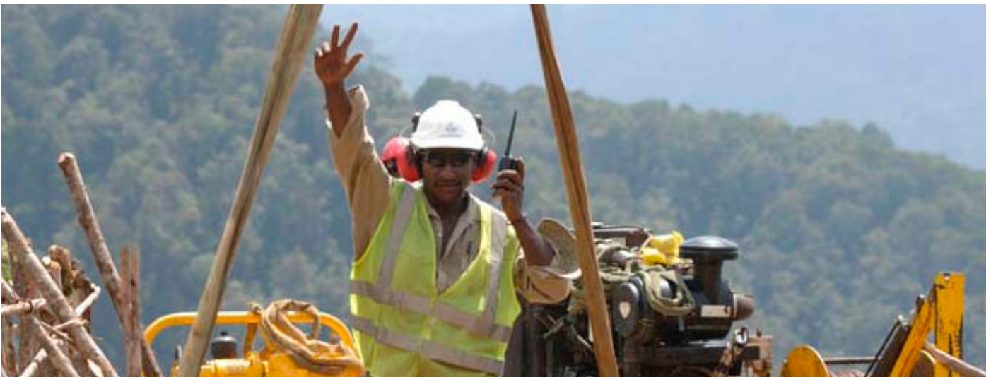
A helicopter supported drill rig move in progress
